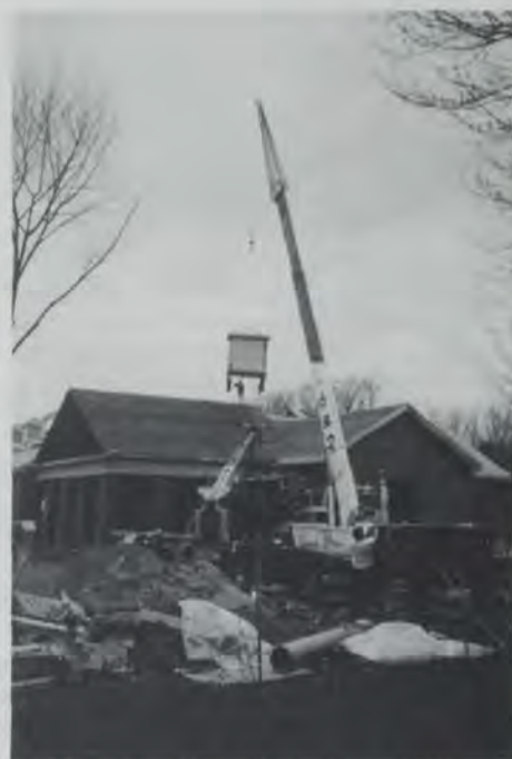
The largest of the nine cupolas is lifted into place.
